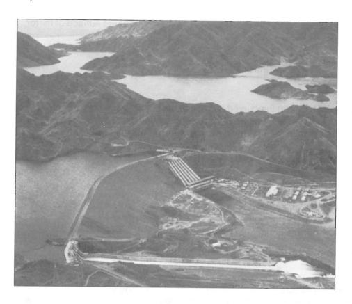
The Benmore Power Station generates 540 MW of electricity for supply around New Zealand. The power station operates by water rushing down the penstocks from the top of a hydro-electric dam to the power station at the bottom. This water then turns a turbine which is connected to a generator causing it to rotate.
